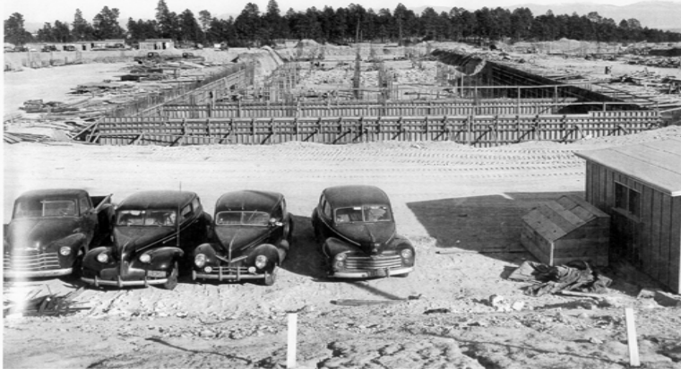
1949 CMR Construction Site
