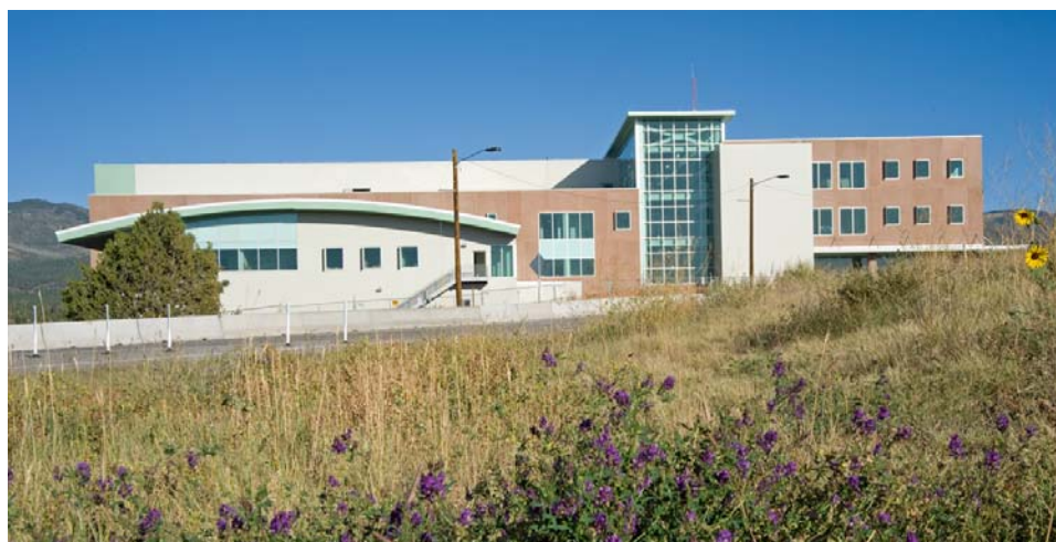
Figure D-9. Chemistry and Metallurgy Research Replacement Radiological Laboratory/Utility/Office Building circa November 2009.
