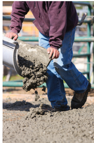
Concrete contains fly ash which lowers the environmental impact and increases durability
