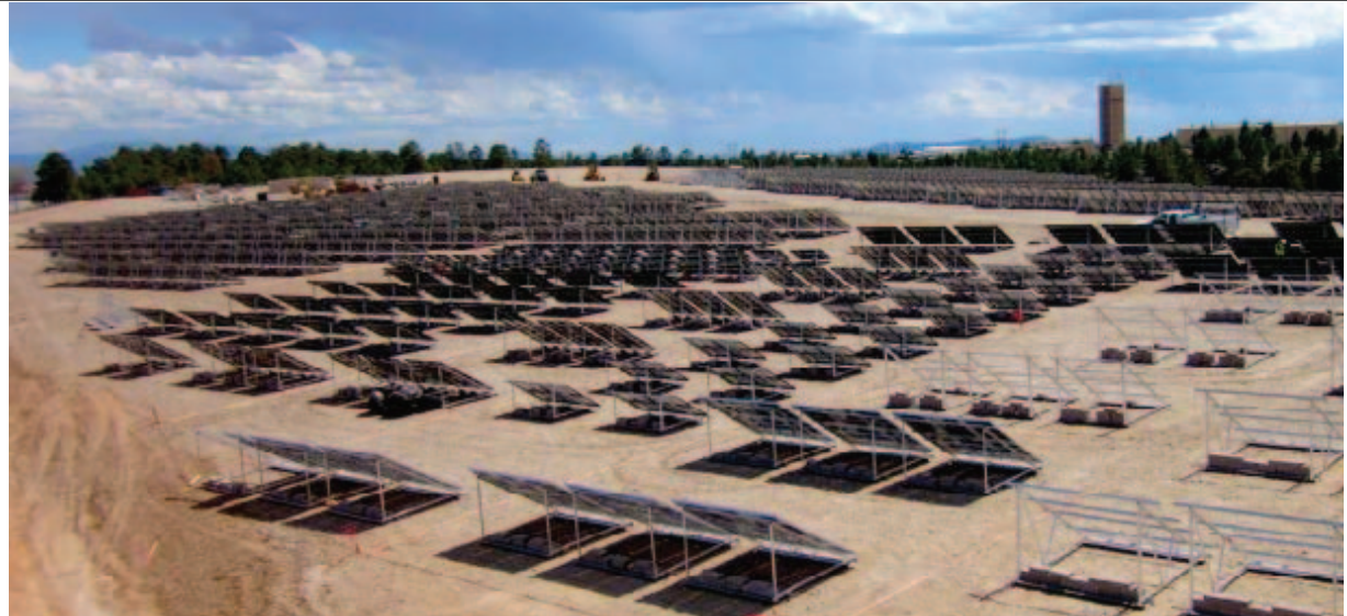
LA County Solar Photovoltaic panels
