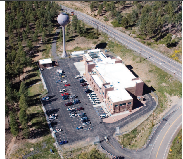
Emergency Operations Center
