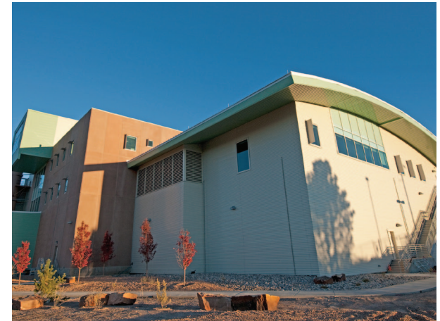
Radiological Laboratory and Utility Office Building
