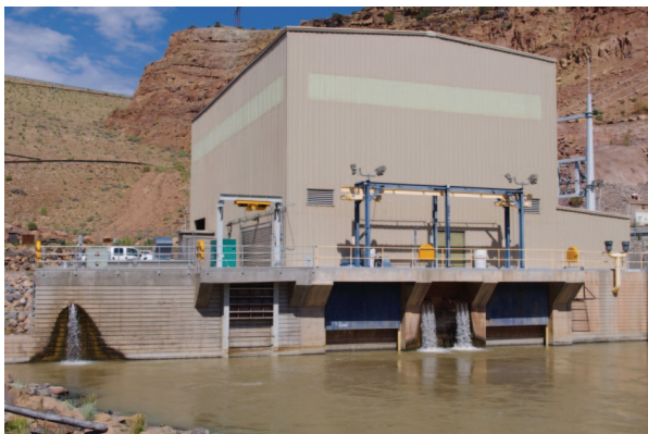
Abiquiu low-flow turbine generator
