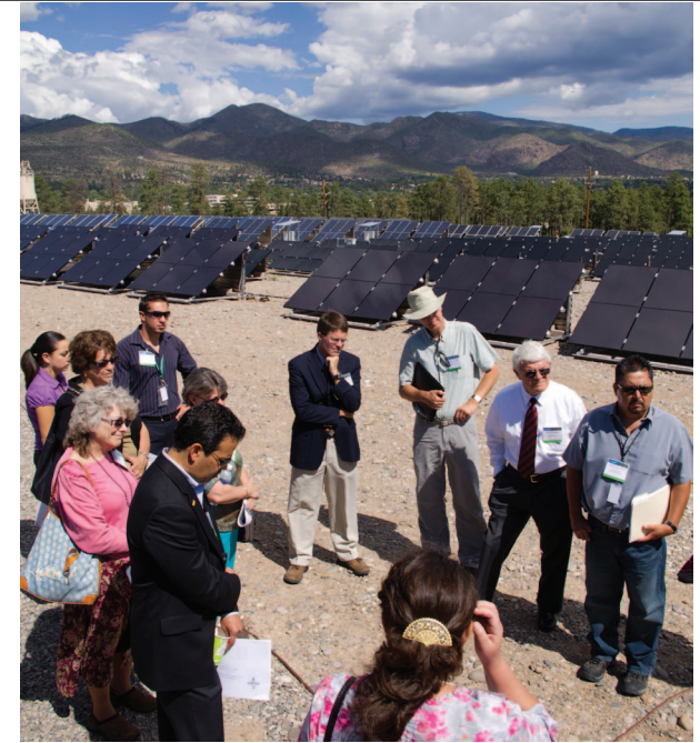
Tour of the Los Alamos County Photovoltaic array
