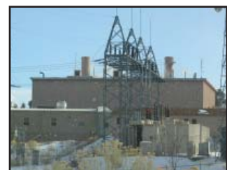
Cogen, TA-3 Steam System Reconfigure
