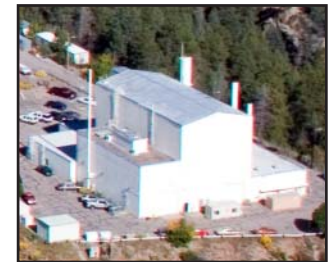
Cold War Era Radiological Laboratory Building at TA-35
