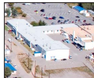
Aging/Obsolete Laboratory at TA-35-0002
