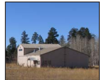
Aging/Obsolete Facility at Fenton Hill
