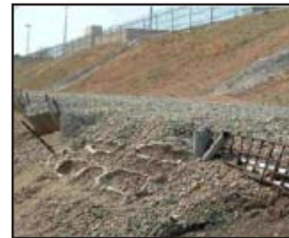
Nuclear Materials Safeguards and Security Upgrades Project (NMSSUP) Phase II
