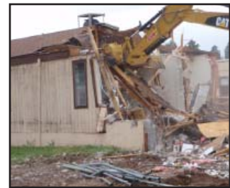
D&D of Temporary Structures
