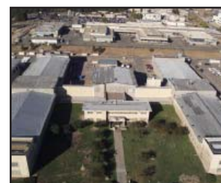
Chemistry and Metallurgy Research (CMR) Facility
