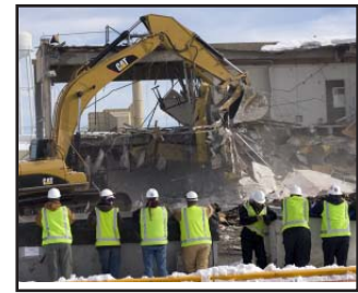
D&D of TA-21 (DP East, West, and the Tritium Systems Test Assembly Facility)
