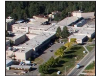
Cold War Era Physics Building (TA-03-0040)
