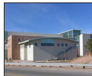
Radiological Laboratory Utility Office Building (RLUOB)
