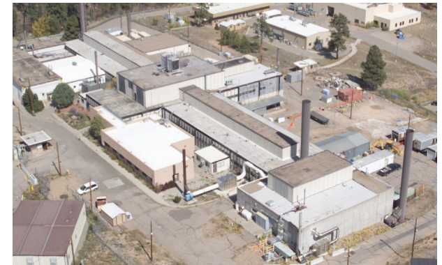
Figure 3.13: RC-1 Life Extension Upgrades.
