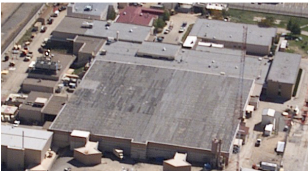
Figure 2.10: PF-4 facility will undergo life extension and seismic upgrades.
