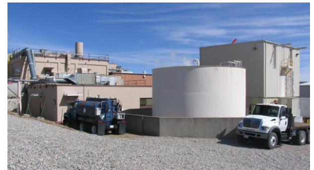
Figure 2.6: Radioactive Liquid Waste Treatment Facility.
