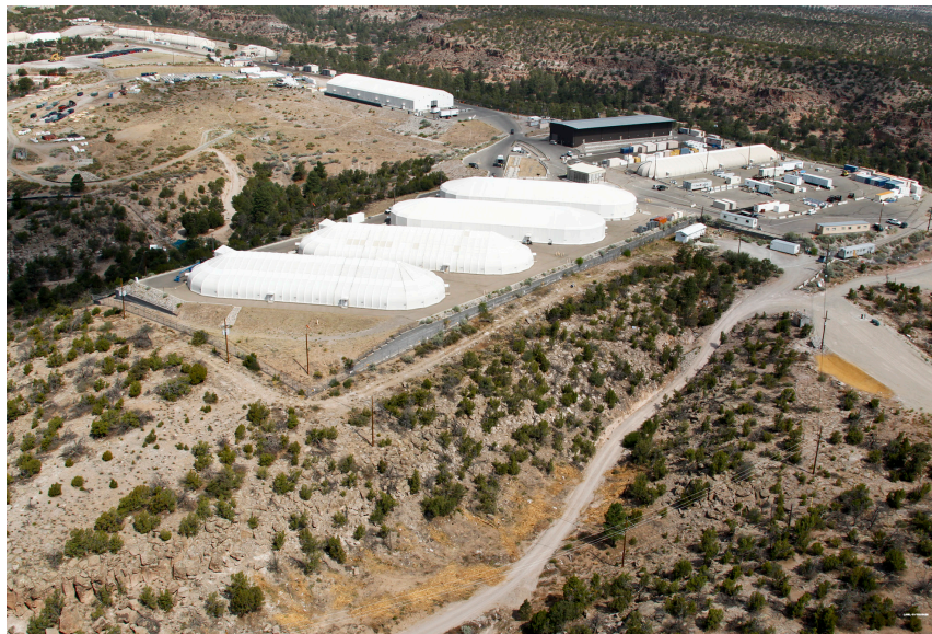
Figure 6.2: Area G storage domes at TA-54.
