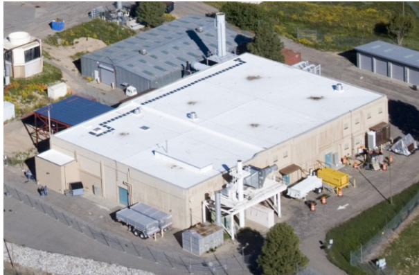
Figure 2.12: Beryllium Technology Facility (BTF).
