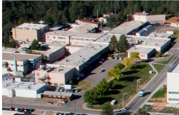
Figure 3.14: Physics building renovations.
