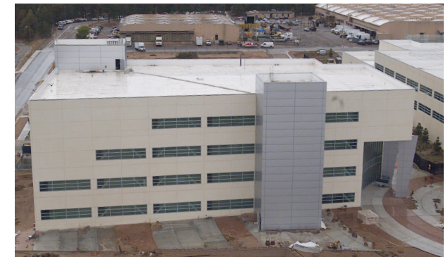
Figure 4.5: Nonproliferation and Internal Security Building (NISC) at TA-3.
