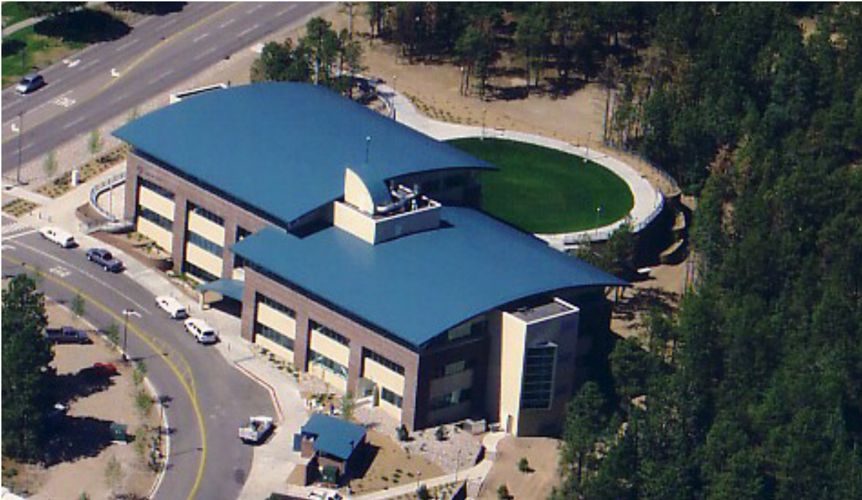
Figure 3.25: Office space within the Research Park is currently being renovated into laboratory space for bioenergy.
