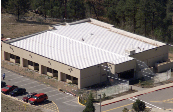
Figure 4.8: Future IAEA Schoolhouse will be located at TA-66 Building 1.
