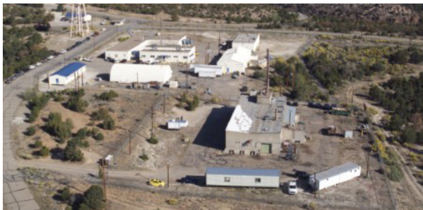
Figure 4.6: Some Global Security activity will continue to take place at remote technical areas, such as the TA-33 Campus, until the Laboratory consolidates to a smaller centralized campus.
