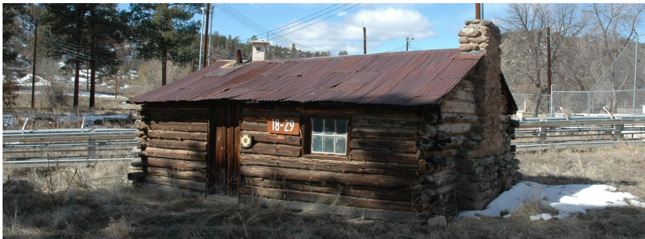
Figure 5.13: The Pond Cabin is a historical structure located at TA-18 and monitored by the Environmental Protection Division.
