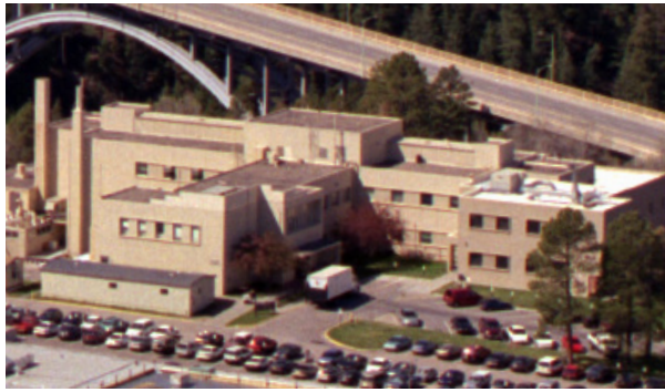
Figure 3.12: Reinvestments to the HVAC system will be necessary for the Health Research Laboratory.
