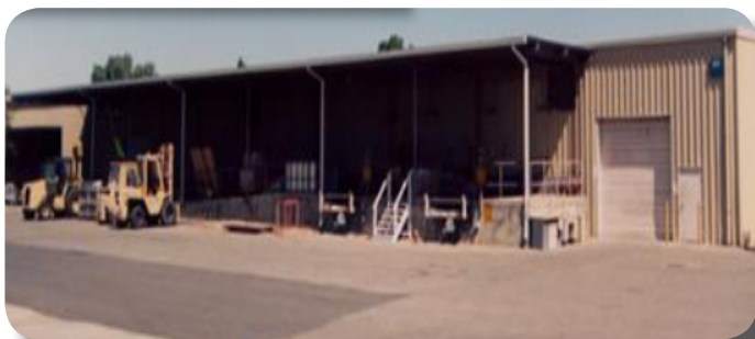
Figure 6.3 SNL/CA Building C927
