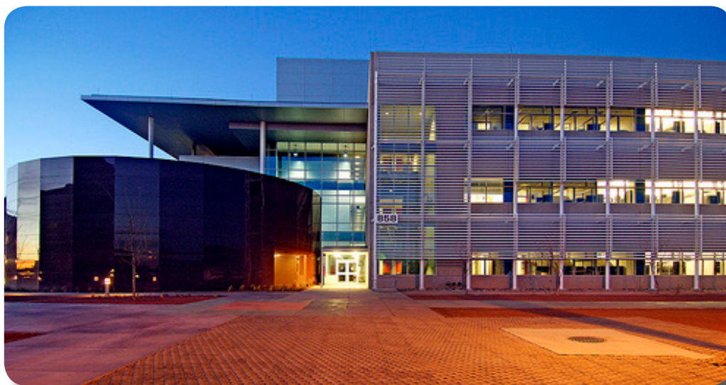
Figure 5.6 View of the MESA Complex from the South
