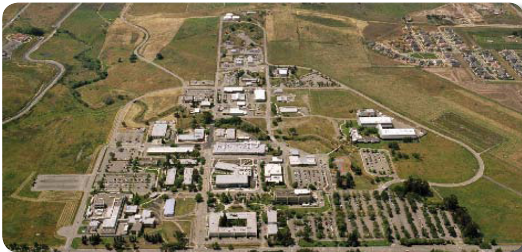
Figure 3.1 SNL/CA Campus, Looking South
