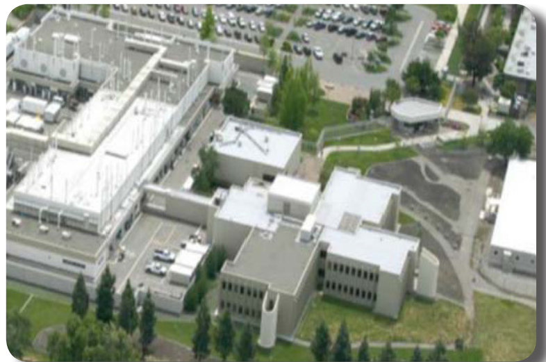
Figure 5.11 SNL/CA Building C905
