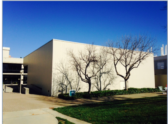
Figure 5.10. SNL/CA Building C904
