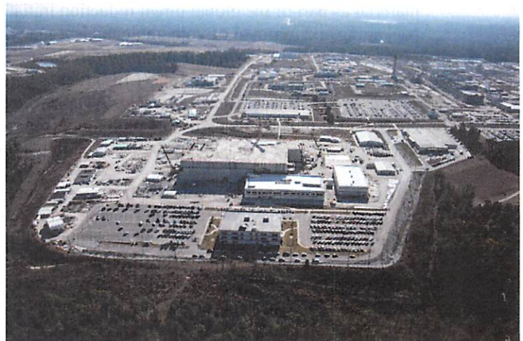
SRS Nuclear Nonproliferation Facilities Under Construction (January 2015)
