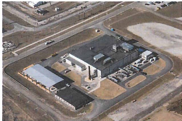
Figure 5-8: Waste Solidification Building (January 2015)
