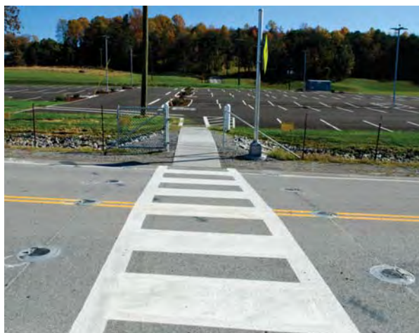
Fig. 2.6. Solar-powered crosswalk at New Hope Center.
