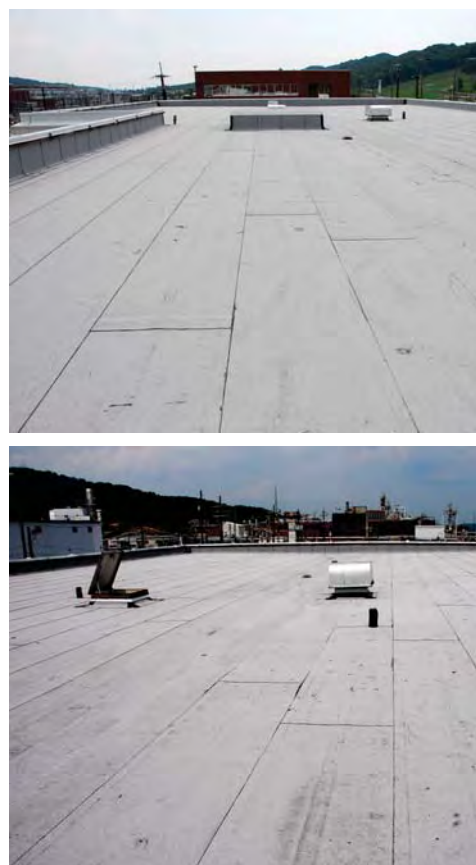
Fig. 2.4. Buildings 9204-02E and 9103 cool roof installations.
