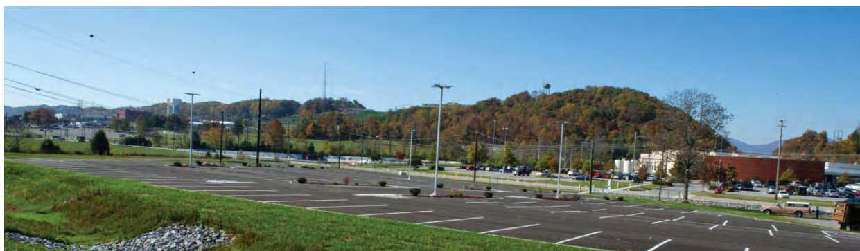
Fig. ES.1. In FY 2012, Y-12's New Hope Center parking lot was constructed utilizing sustainable products and techniques
