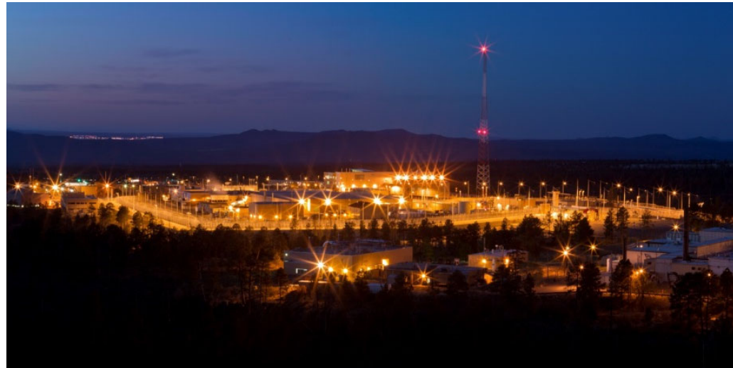
Plutonium Facility within Technical Area 55
