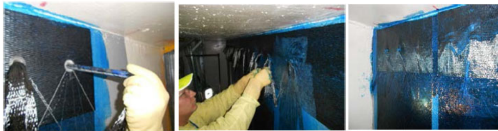
Reinforcing Roof Girders with Carbon Fiber Wrap
