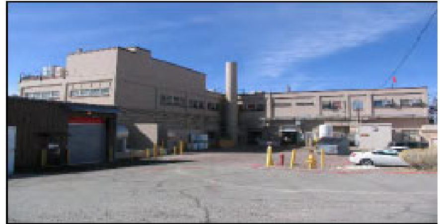
Existing Radioactive Liquid Waste Treatment Facility
