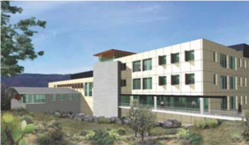
RLUOB as viewed to the Northwest
