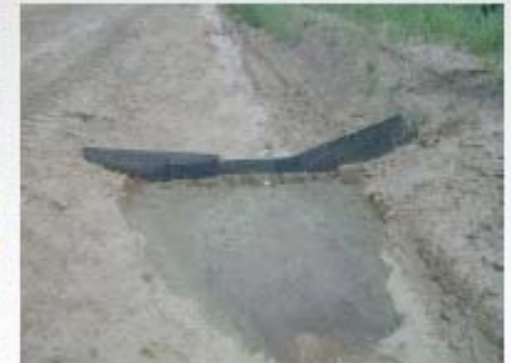
Georidge™ panels for runoff control and sediment transport.
