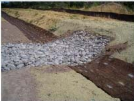
Turf reinforcement mat and rock for erosion protection and energy dissipation.
