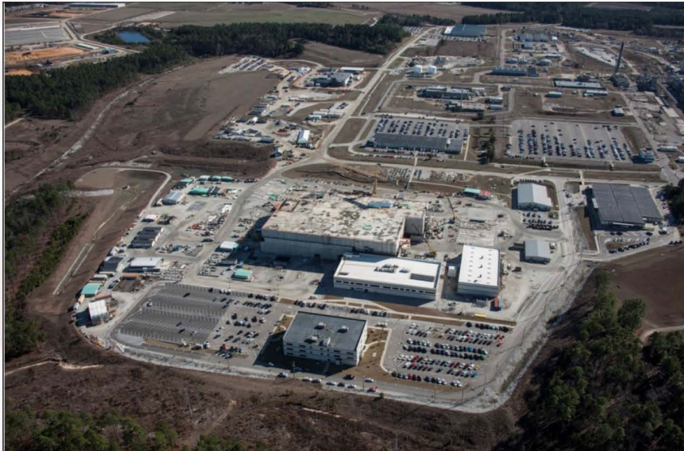
Figure 1: Aerial View of the Mixed Oxide Fuel Fabrication Facility Construction Project
