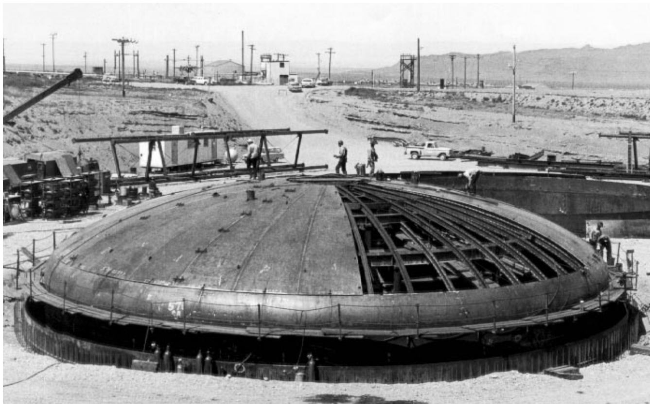
Figure 1.2: Construction of Double-Shell Tank at Hanford
