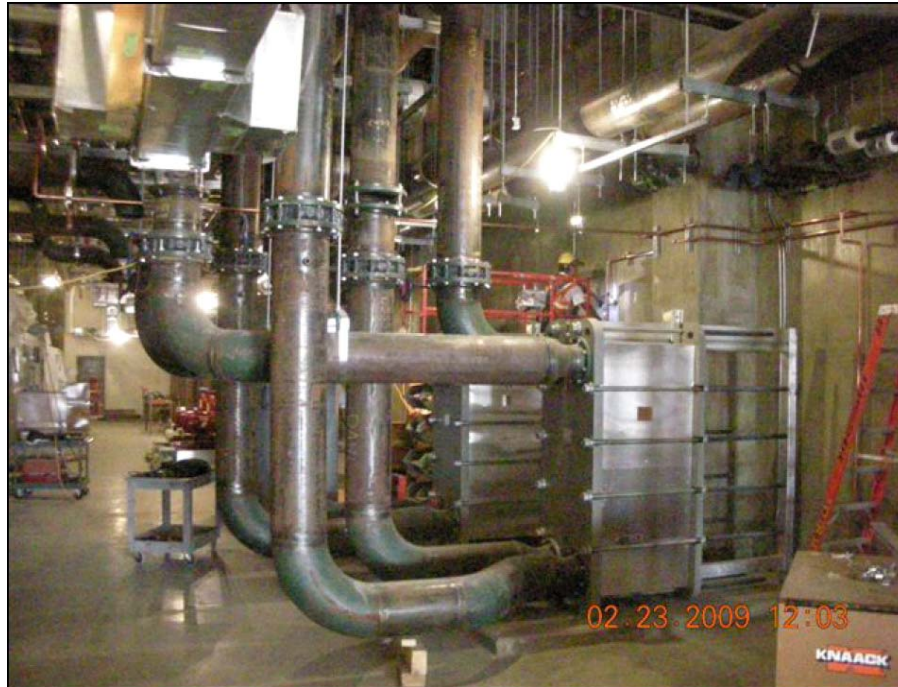
1 st Floor Central Utility Building – Installation of Heat Exchangers and Pumps
