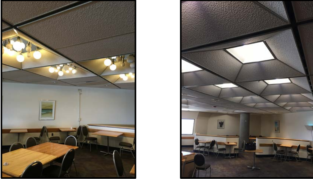
Picture 2. LEDs linear lighting-Before and after in main Cafeteria
