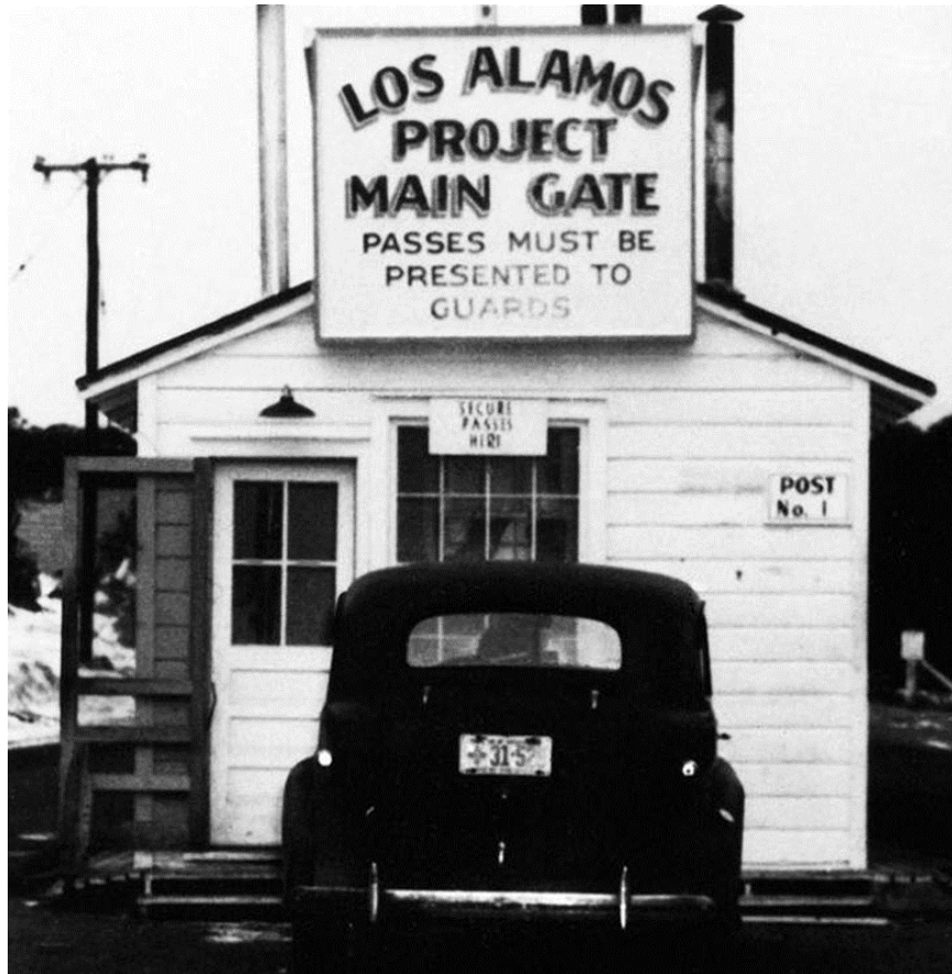
Figure 4-A: Photo of the original Los Alamos Project Main Gate
