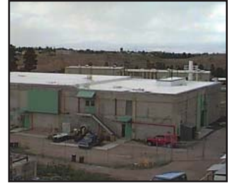
Beryllium Technology Facility (BTF)
