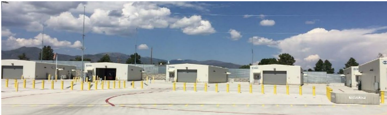
Figure A.2.2-7 Transuranic Waste Facility at LANL
