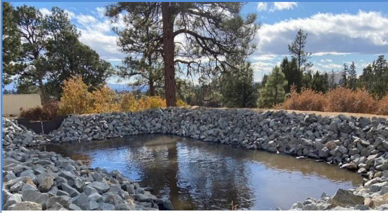
TA-35 Parking Lot Basin Low-Impact Design (LID) Landscape Project
